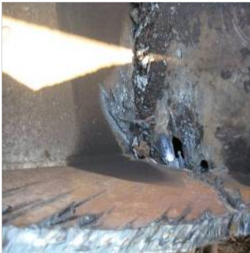
Figure 1. Damage to stacker unit from detonator explosion
